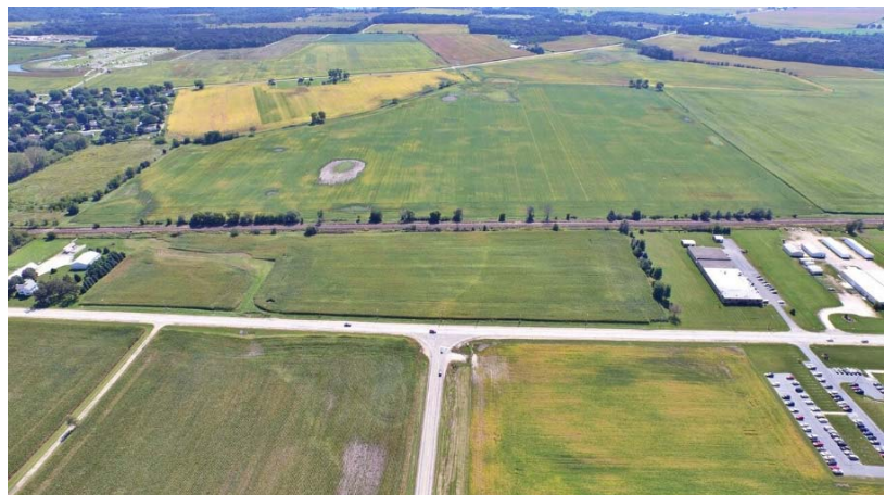
Intersection of Dauberman Road and US Route 30 looking south
